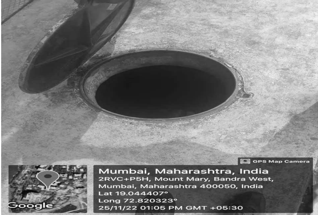
Underground rain water tank
